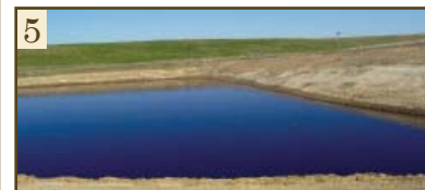
Runoff evaporation pond collects dirty water running off lots and is designed to evaporate a portion of the collected water.
