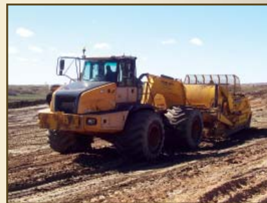
Excavating a runoff containment pond
